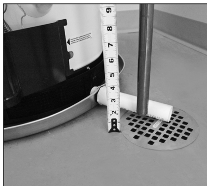
Figure 26 - Temperature and Pressure Relief Valve Pipe
