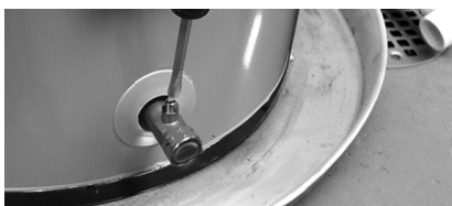
Figure 42 - Draining the water heater.
