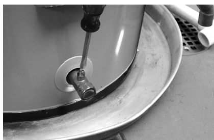
Figure 20 - Draining the old water heater.
