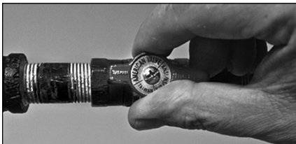
Figure 32 - Gas valve in "on" position
